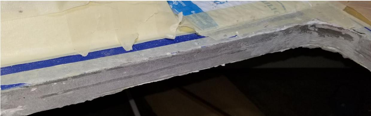
After Bondo fiberglass cloth with fiberglass resin
